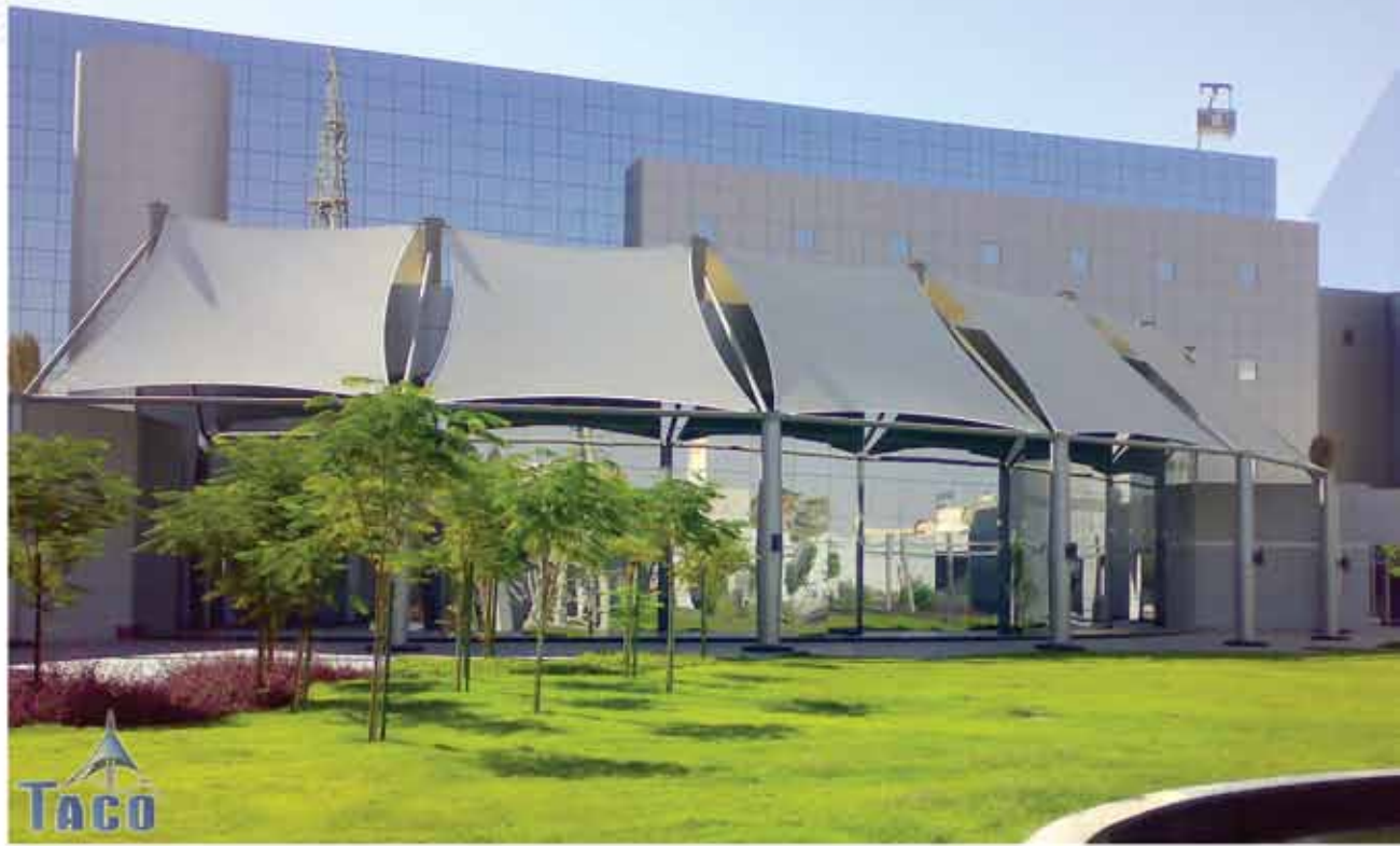
Al Jawal Building Tent-STC
