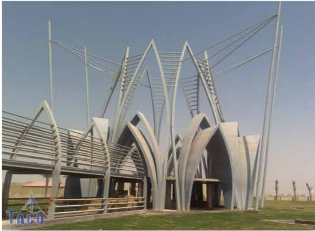
Tension Steel Structure Awning – Private palace
