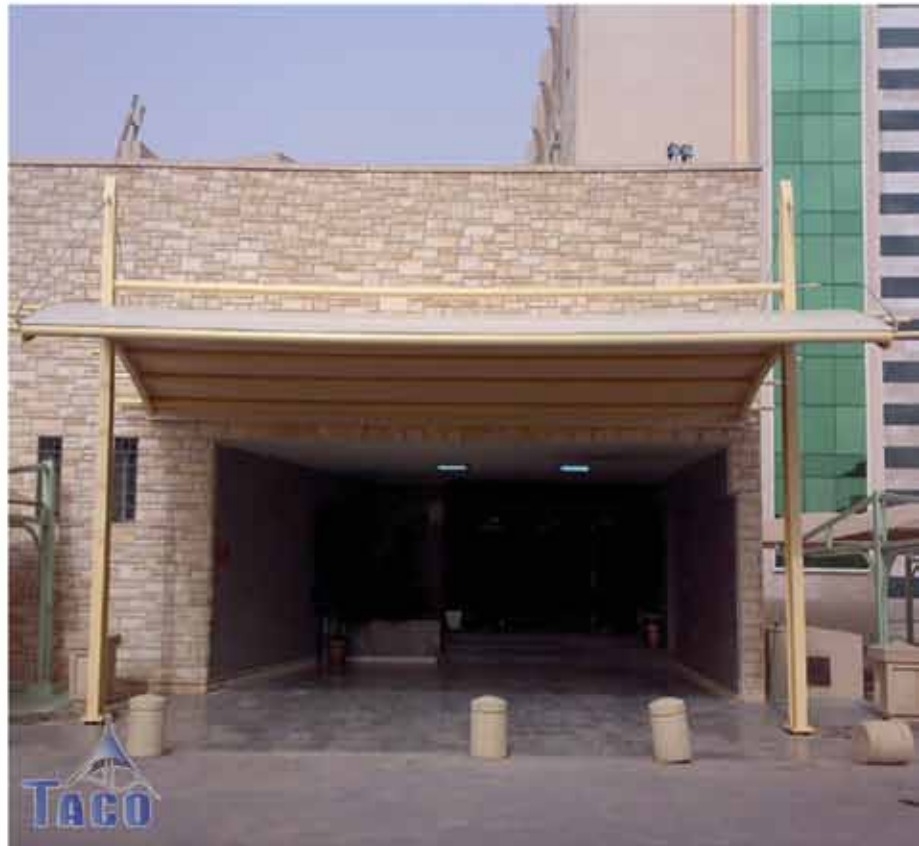
Courtyards and Entrance Awning- Ministry Of Education
