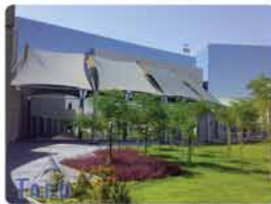
30 - Entrance tension structure awnings
