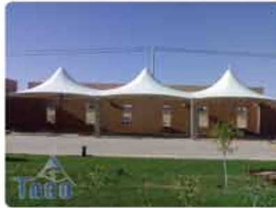
6 - Continues conical awnings
