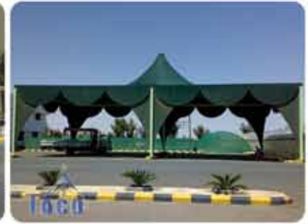
23 - HDPE Awning for sitting area
