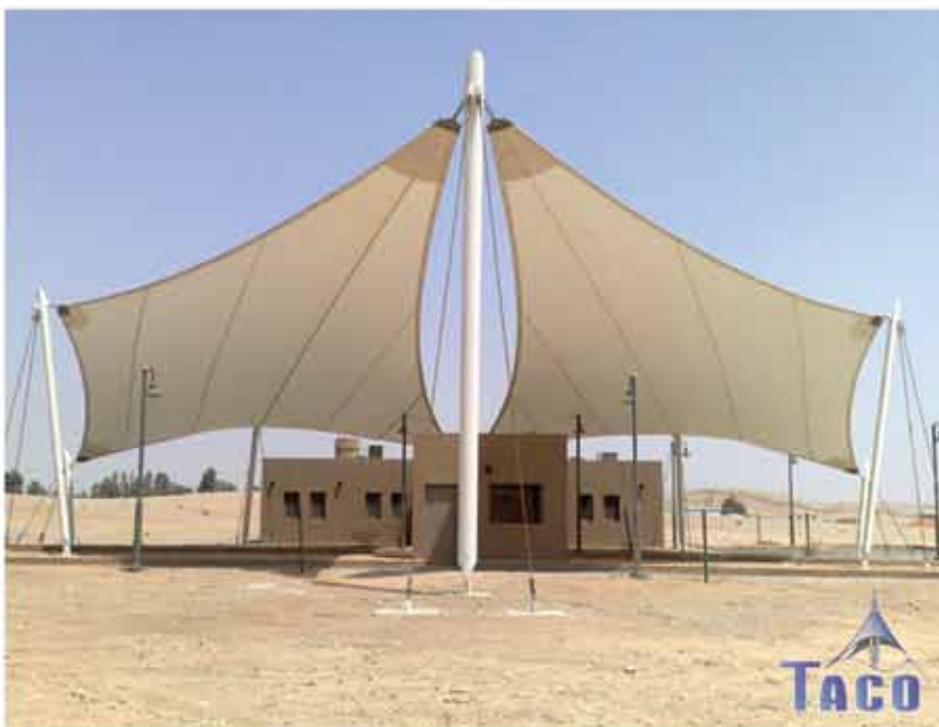
PanPan Garden resort – Entrance Awning - Main Gate
