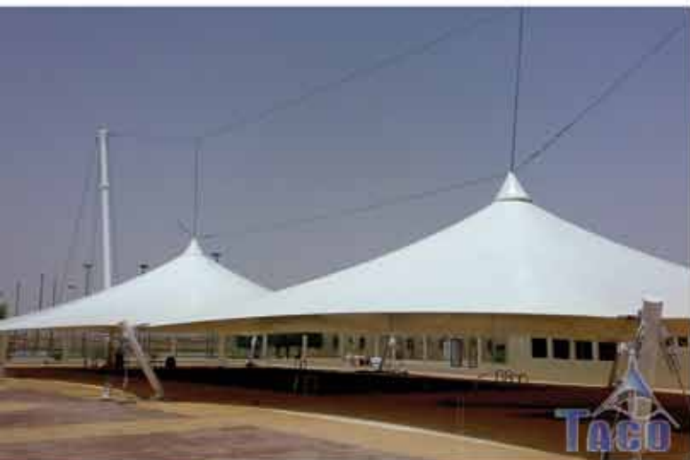
Swimming Pool Awning – Qassim cement factory
