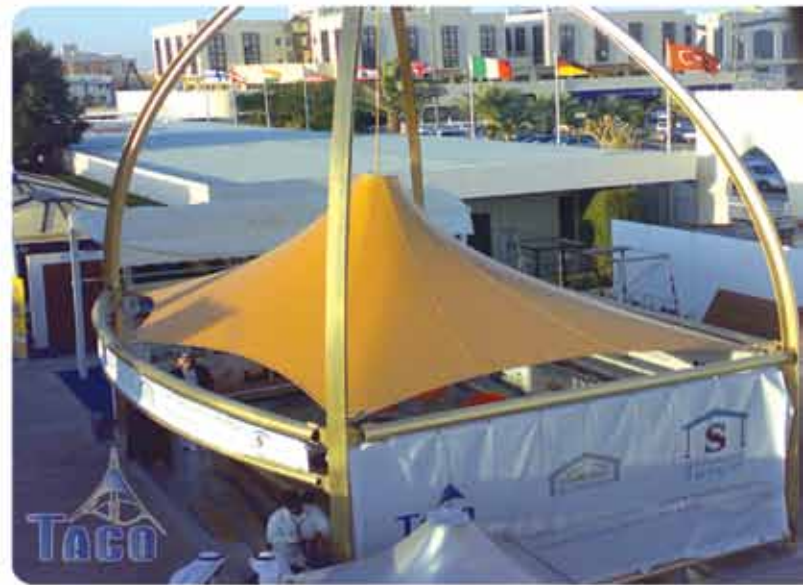
11 - Conical awning tensioned by beams
