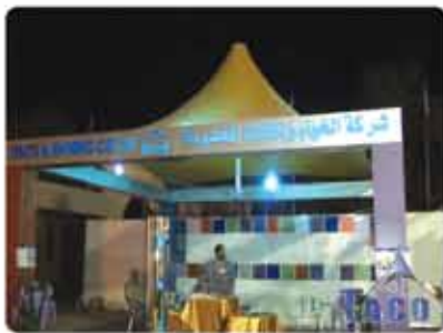
12 - Tensioned conical awning with push up cables
