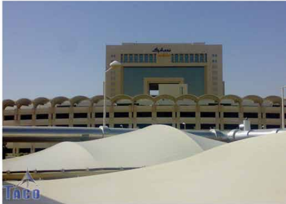
Chiller Area Awning- SABIC HQ Riyadh
