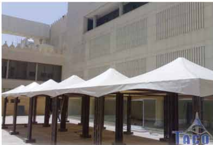
Governorate of Deera Building's Awnings
