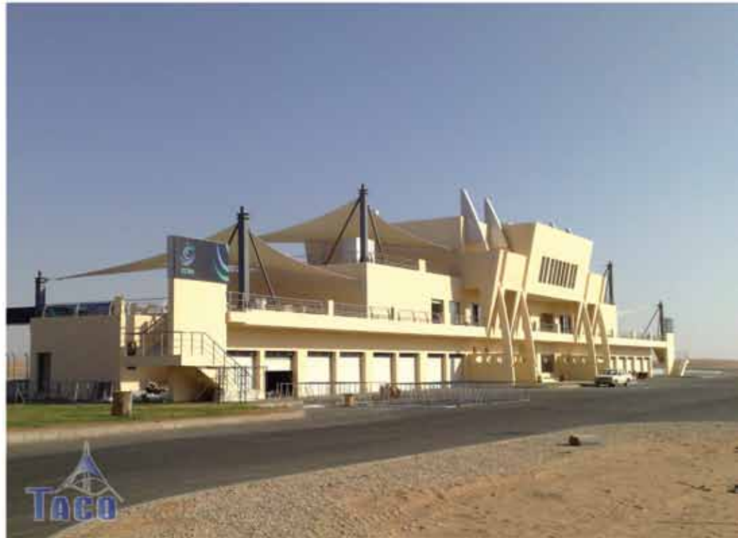
Al-Reem Car Race – Main Building – Tension Fabric structure
