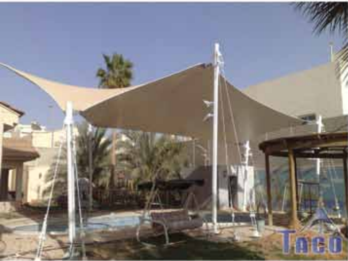
Tension Structure Awning Special Swimming Pool
