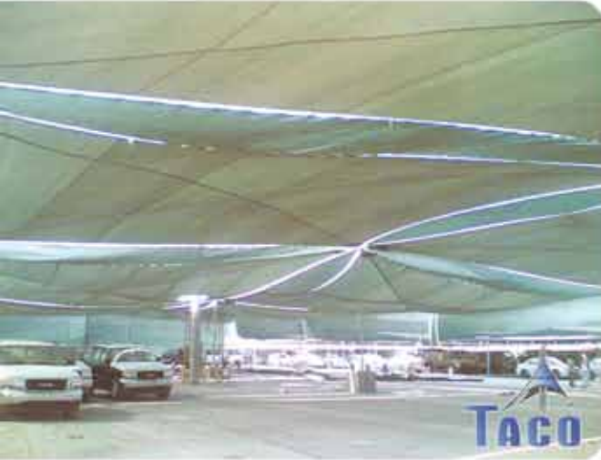
45 - HDPE tensioned fabric awning
